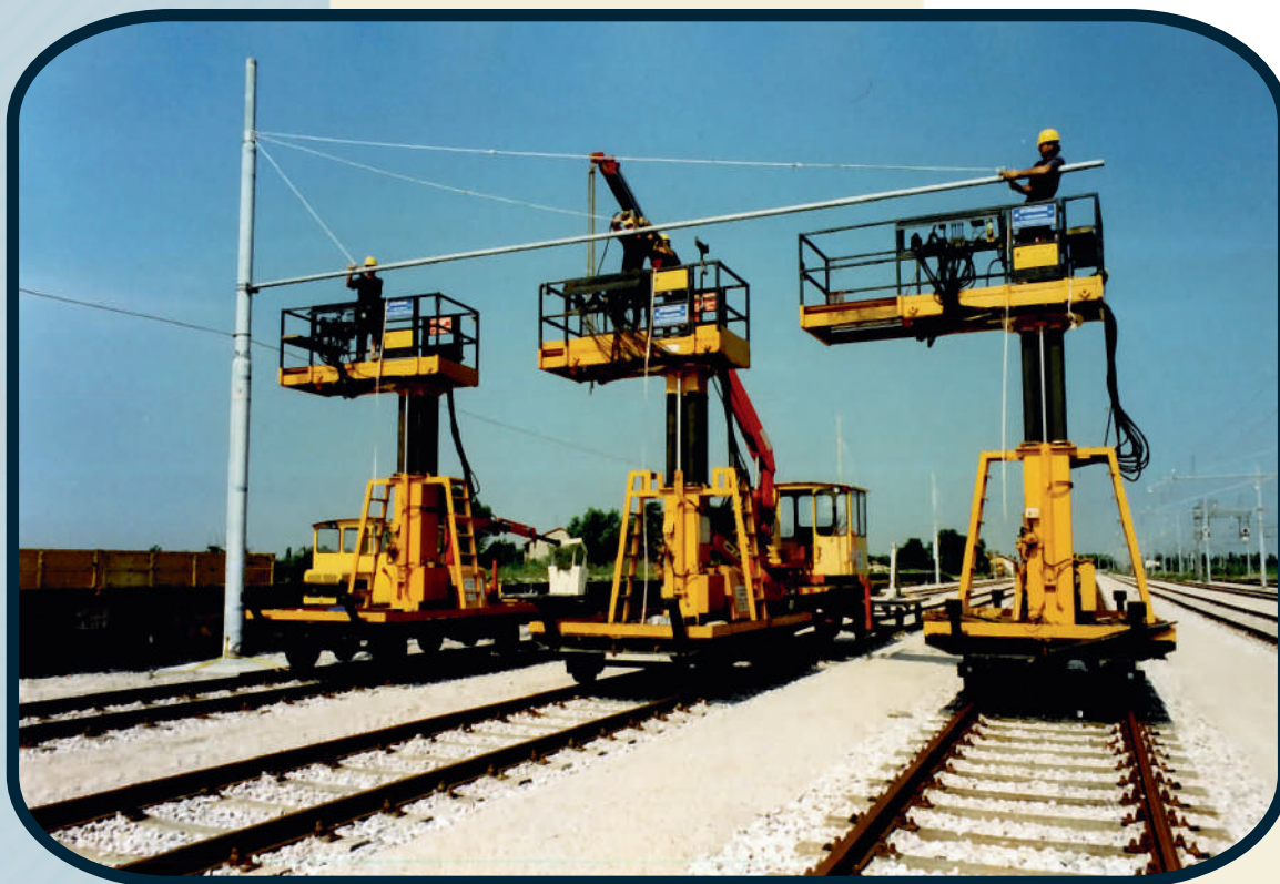
Villa Vicentina (UD), 1986 Laying of cantilevers on three tracks
