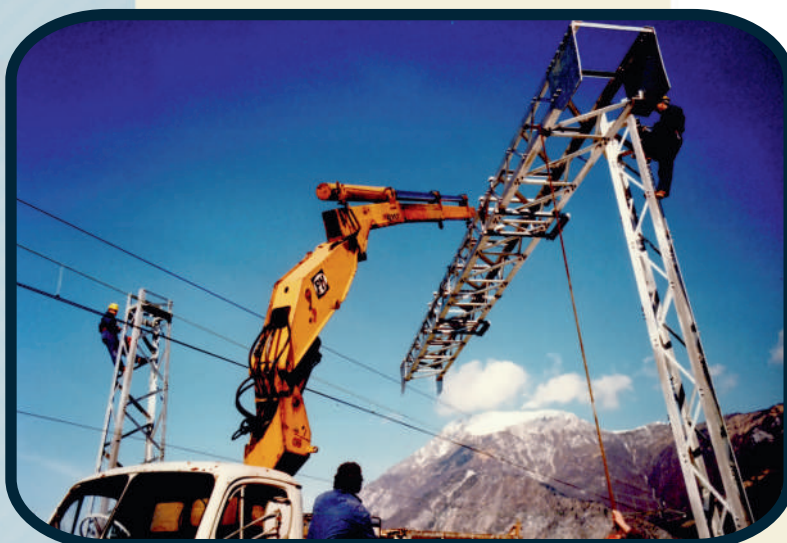
Carnia (UD), 1992 Laying of a station gateway
