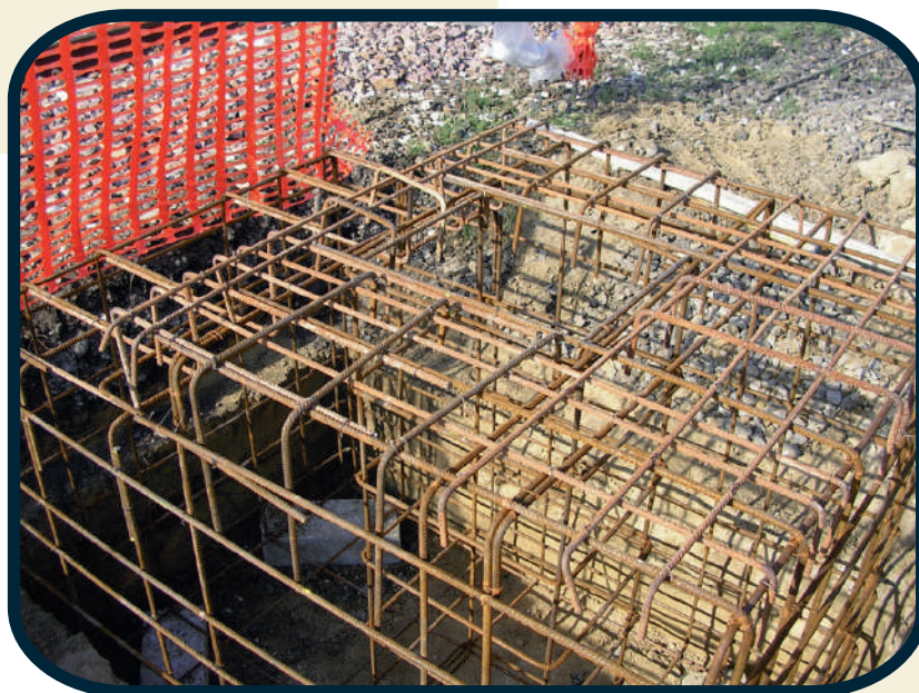
Vigonza, 2005 Reinforcement concrete blocks
