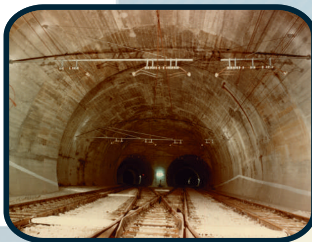
Trieste, 1980 Electrification of the belt tunnel
