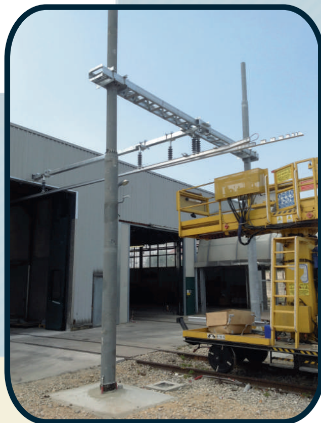
Vicenza, 2013 Electrification of the track n ° 10 at the Workshop of Cyclic Maintenance (OMC) ETR
